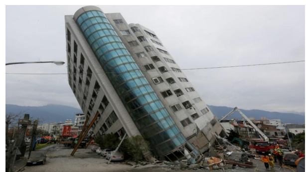
Fig.2 Damage of building because of earthquake
