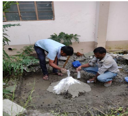
Fig-1. Mixing of glass powder and copper slag in concrete
