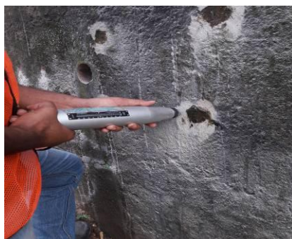
Fig -4: Rebound Hammer Test.
