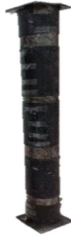
Fig 4. Column after application of load
