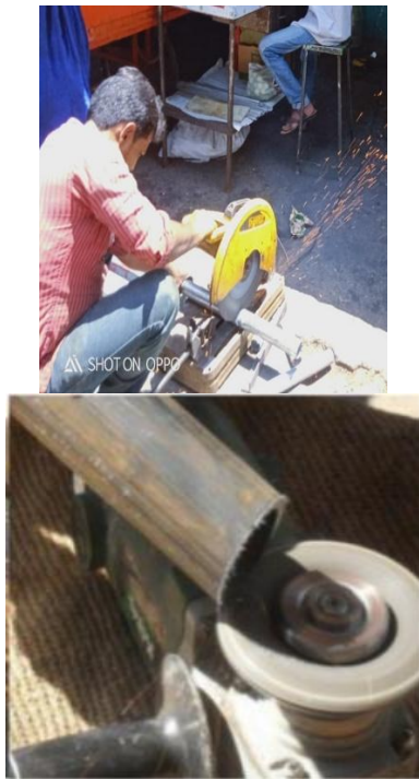
Fig 4.1.1 Cutting of galvanized steel tubes and Pruning the edges
