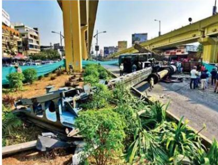
Image 2: Pune Metro Pillar Accident. Source: Times of India
