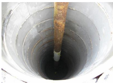
Figure 2: Dangerous Borewell Hole
