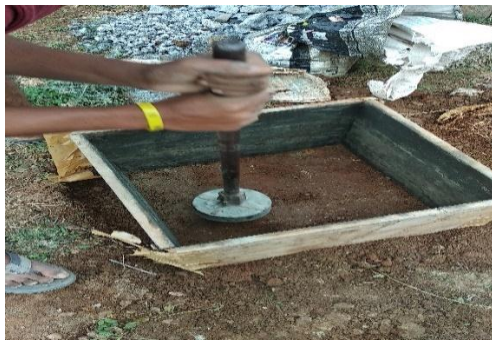
Figure -2: Subgrade preparation
