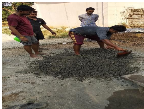
Figure -3: Mixing of constituents
