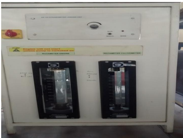
Fig: Water flow measuring rota meter.
