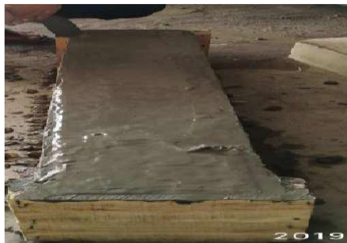
Fig (2.5) After Concreting the Formwork
