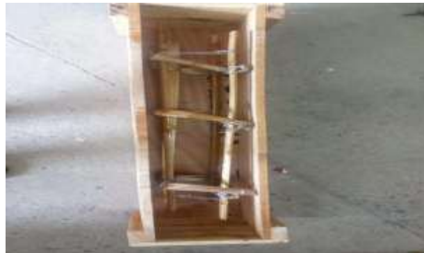
Fig (2.3) Formwork preparation before concreting
