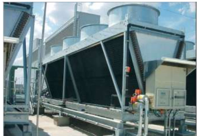
Figure 15 Hybrid Dry Cooler
