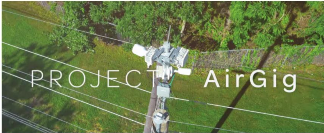
Fig. 4. Aerial view of Project AirGig node.
