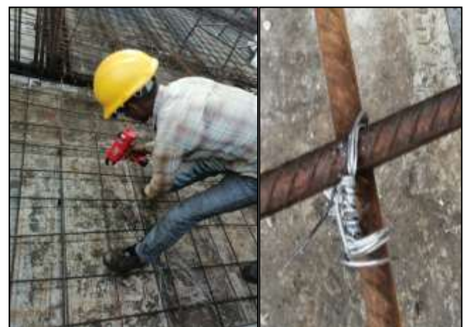
Fig.5 Labor using rebar tying machine on site and enlarged image of a knot by the machine
