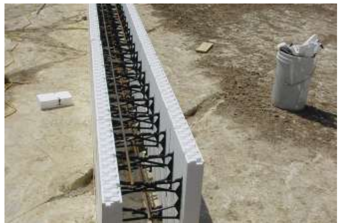
Fig -3: ICF Blocks
