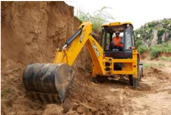
Fig -1: Excavators (JCB)
