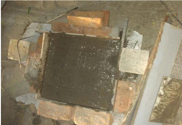
Fig. 13: Green Slab Just After Finishing
