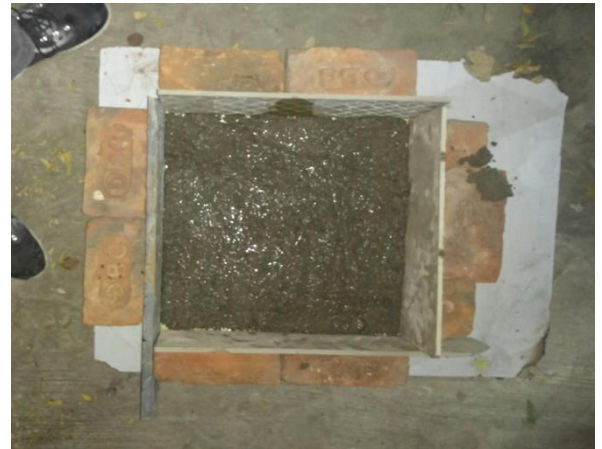
Fig. 11: Placing Of 1 st Layer of R.C.C. 20mm Thick
