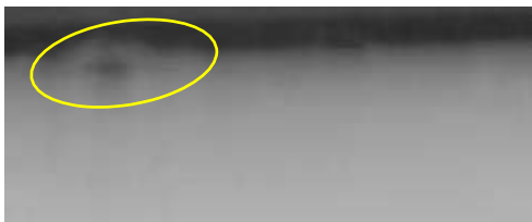
(c) Outer ply delamination
