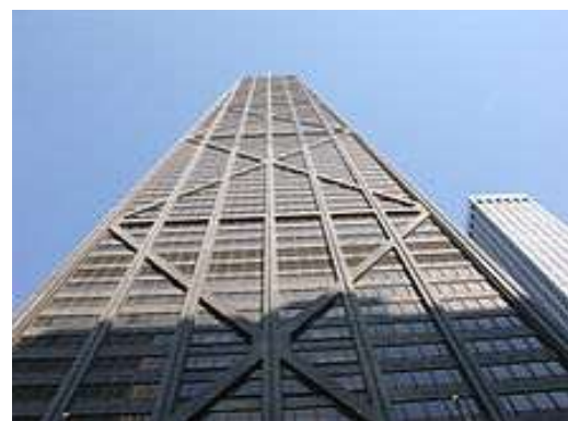
Figure: 1.1 Cross Bracing.
