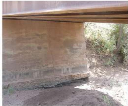
Fig: Differential Settlement Under an Abutment Drilling and plugging
