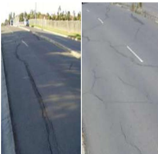
**Cracking and pavement damage on western approach**
