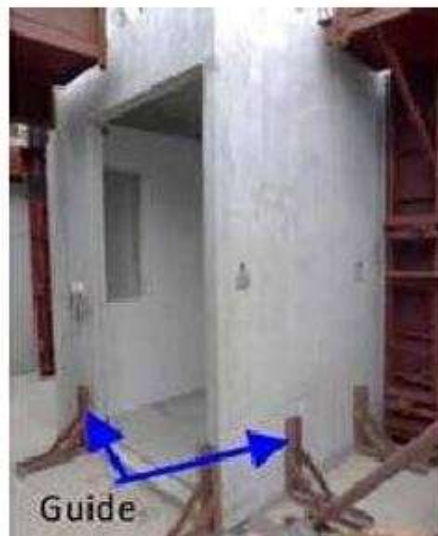
Fig -1.4: Positioning PBU
