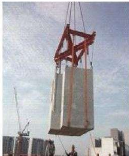
Fig -1.3: Lifting of PBU at site
