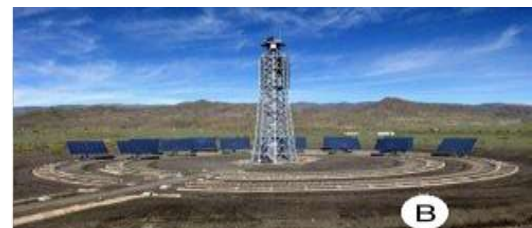
Fig: Central receiver with variable Geometry at CTAER [32].
