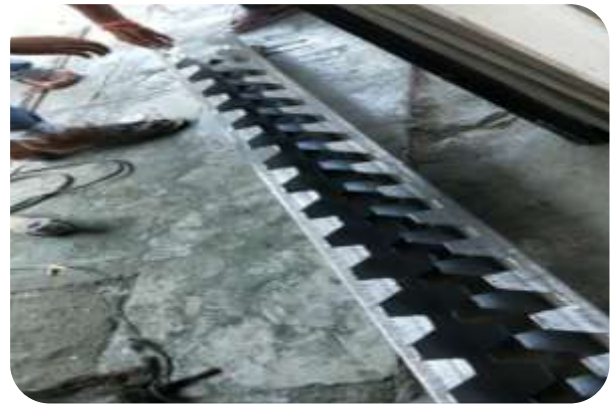
Fig -2: Rearranging and welding the section
