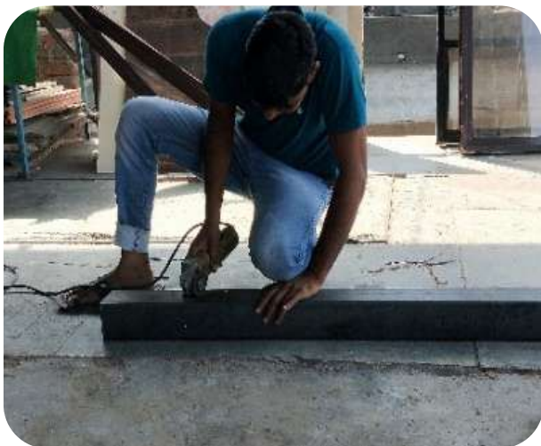
Fig -1: Cutting of Hollow column
