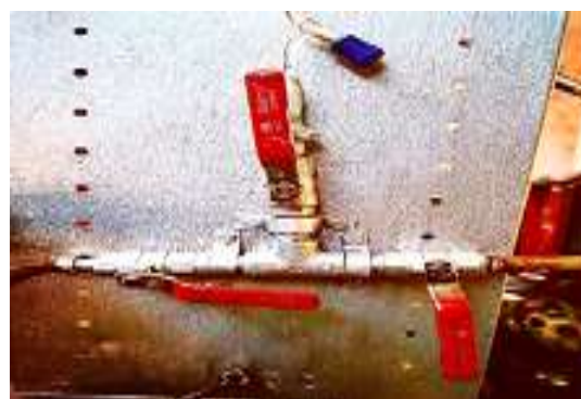
Fig -5: Panel board with valves and burette
