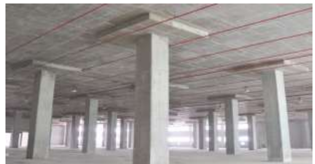
Fig -1: Flat slab with Drop Panel
