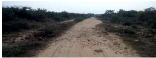
Figure 1.2: Existing Road Surface
