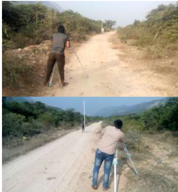
Figure 3.1: Field Surveying for Taking Levels
