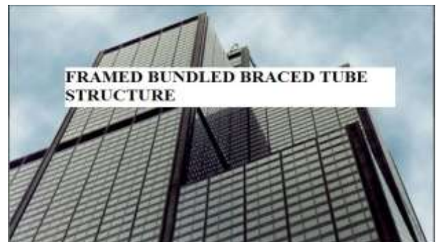
Fig 1.0 Framed bundled braced tube Structure
