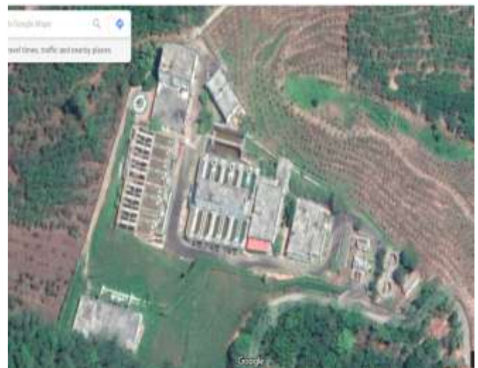
Fig-1 Aerial view of water treatment plant Panamkuttymala, Punalur, Kollam
