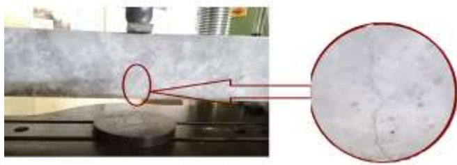
Fig -13: Beam Cracking
