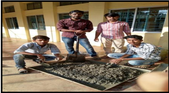
Fig. 4 (Mixing Concrete)
