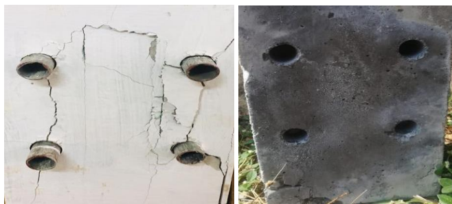
Fig -5: Failure mode of steel specimen (S1)
