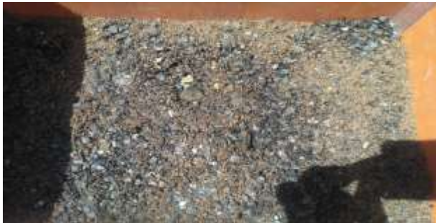
Fig 8 Shows Layer of Coarse Aggregate
