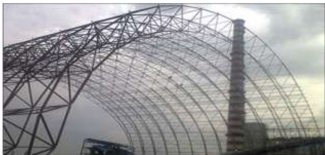
Fig 1 Double layer steel braced barrel vault structure
