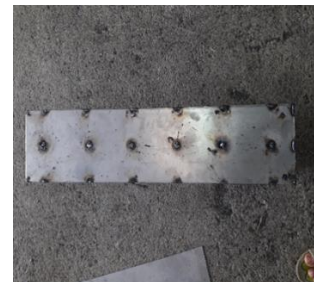
Fig 5: Welded Connection at flange
