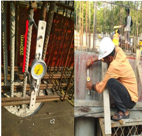
Fig -3: Gauge Distance at Main Reinforcement Bar
