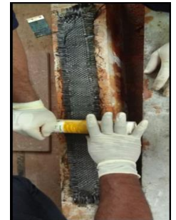
Fig-7: Bonding CFRP
