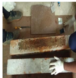
Fig-6: Application of Epoxy
