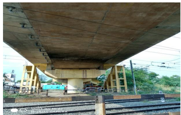
Fig -4.2: Structure of bridge under the railway track
