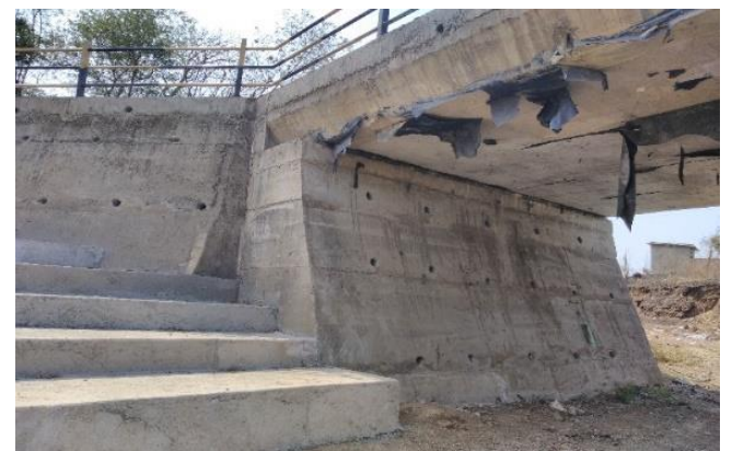
Figure 1.2 Gravity wall cross section on site
