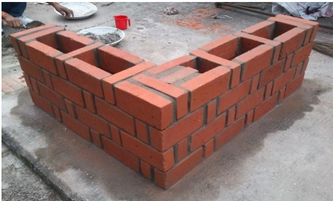
Fig.1 Typical picture of Rat-Trap bond
