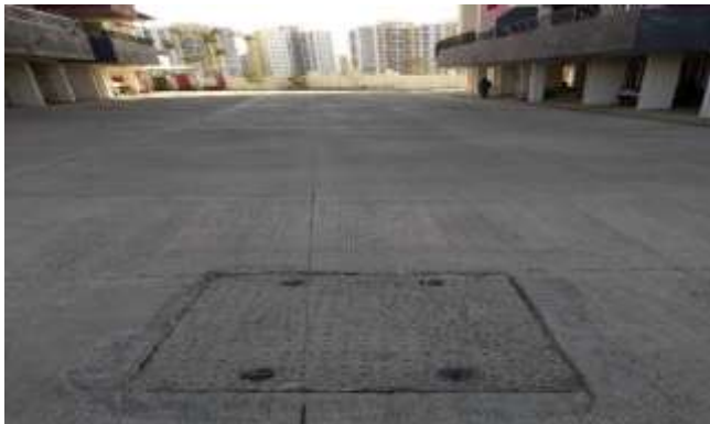
Fig.3- Underground pipe Drain
