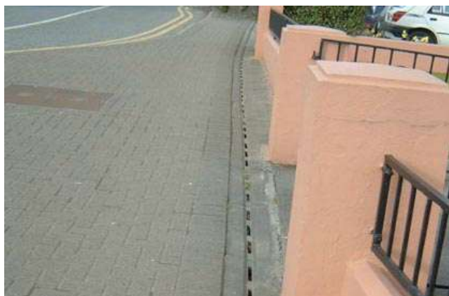
Fig.4 Line Drainage Channel
