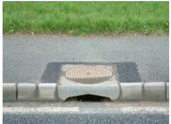
Fig.5 Side entry Gully
