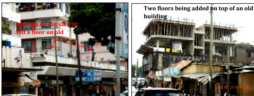
Figure 5: Vertical extension along Sikukuu and Kirk Streets
