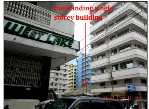
Figure 4: Demolition of old Swahili
