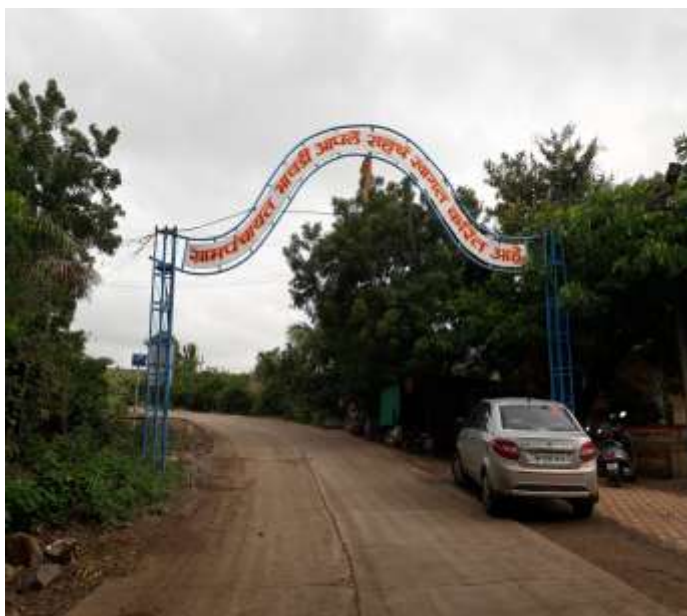
Fig -2: Concrete Road
