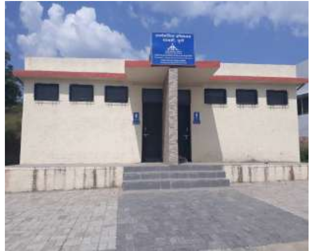
Fig -6:Public Toilets
