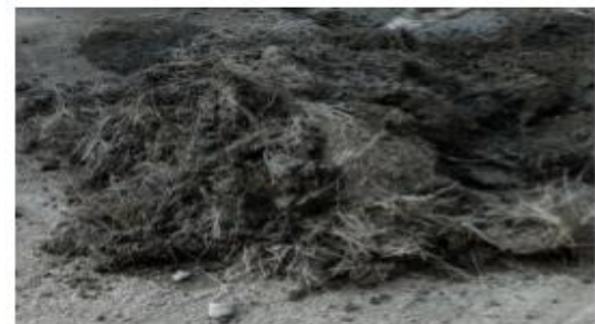
FIG: 1.2 MIXING OF ECC CONCRETE
