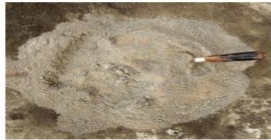
FIG: 1.MIXING OF ECC CONCRETE
