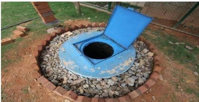
Fig - 3: Recharge well
