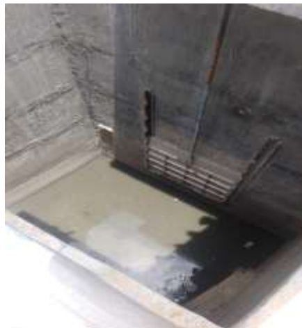
Figure 1: Inlet of 20MLD STP in Davanagere
