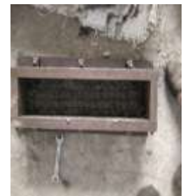
Fig -2: Geogrid placing on beam
