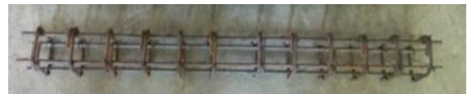
Fig-1: Reinforcement cage for beam specimen
