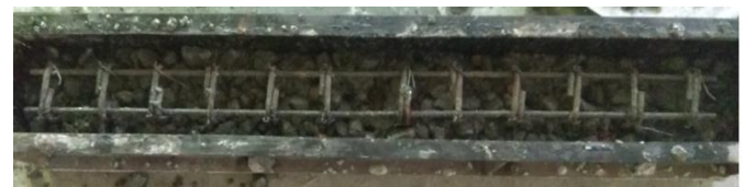
Fig-2: Casting of replaced beam
