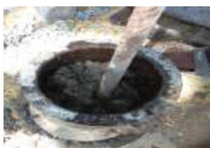
Fig. 5: Casting of Cylinder.
