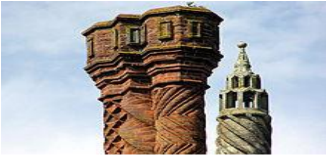
Fig 3.1: Carved brick chimneys characteristic of late Gothic Tudor buildings, at Thornbury Castle, 1514
