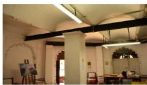
Vaulted slab resting on an I-Section
