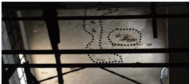
Development of crazing in the slab
