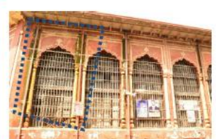
Water leakage through pipes
