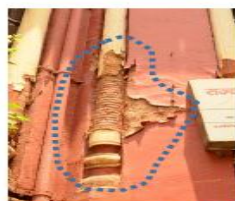
Partial expose of brick work
