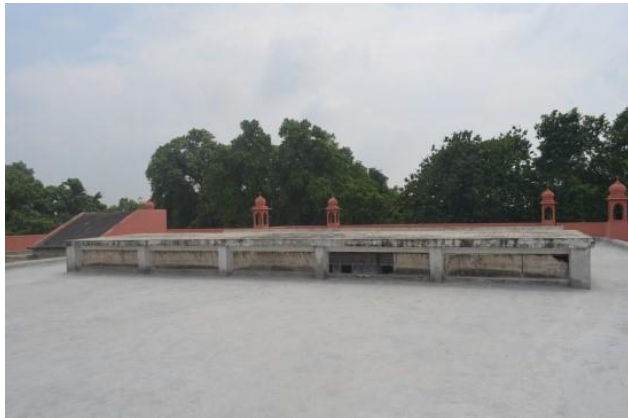
Fig 8: Roofs, Lal Baradari
