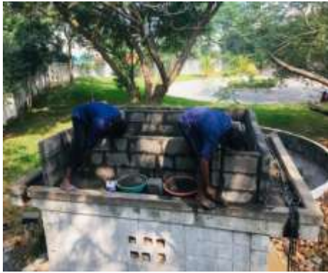
Fig-1 Parapet Construction
