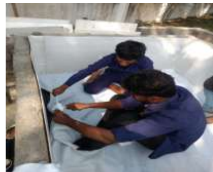
Fig-4 Laying of filter media
