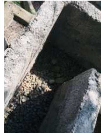
Fig-7 Setting up of Drainage Layer.
