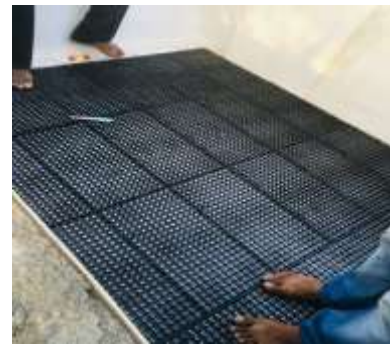
Fig-3 Laying of Drainage Mat
