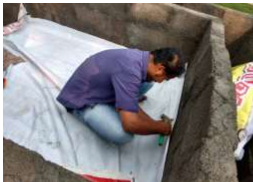
Fig-2 Laying of impermeable membrane
