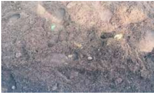
Fig-5 Laying of Growing Media
